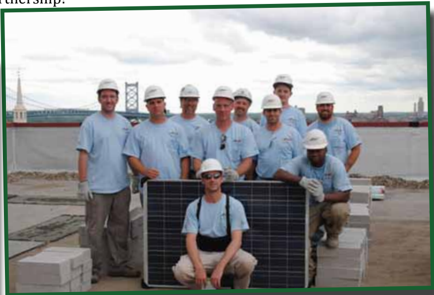
98 Electricians beginning the Solar Panel installation at the Bourse.
